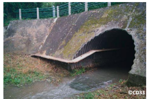
A wooden plank path allows the mink to follow the stream without having to step onto the road.
